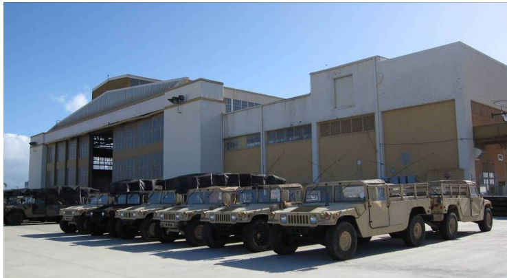
Kalaheo – Maintenance and Repair Hangar. Built 1944.
