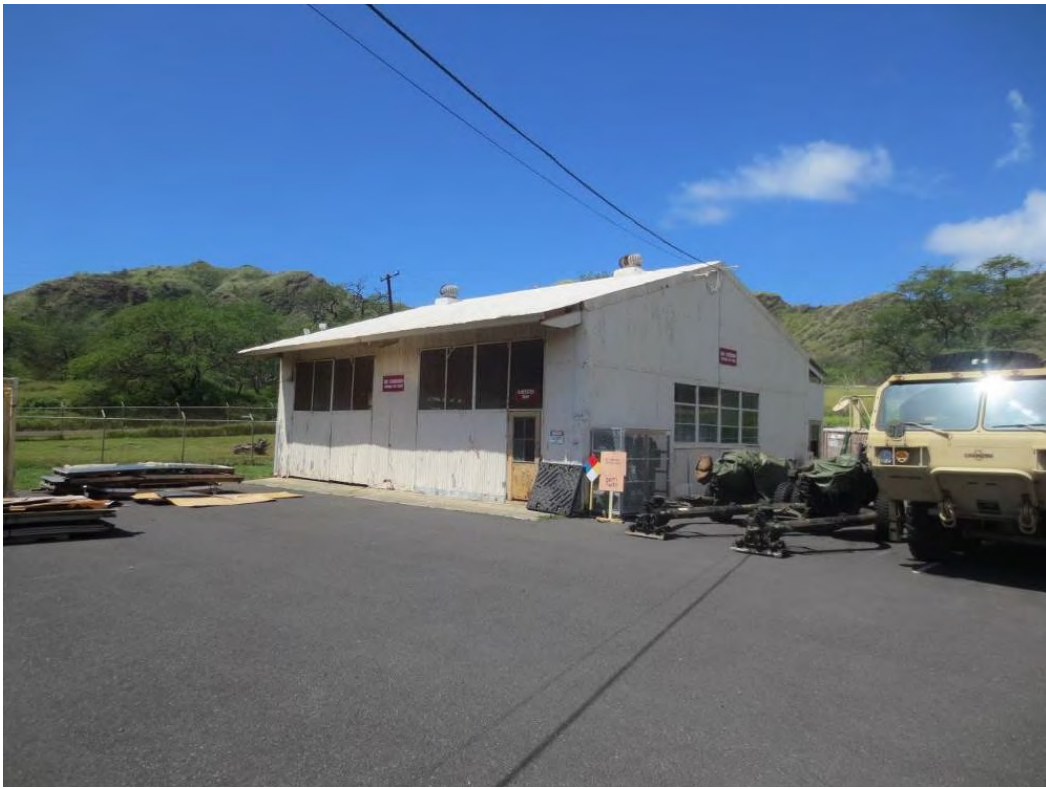
Bldg 304D Front Facade
