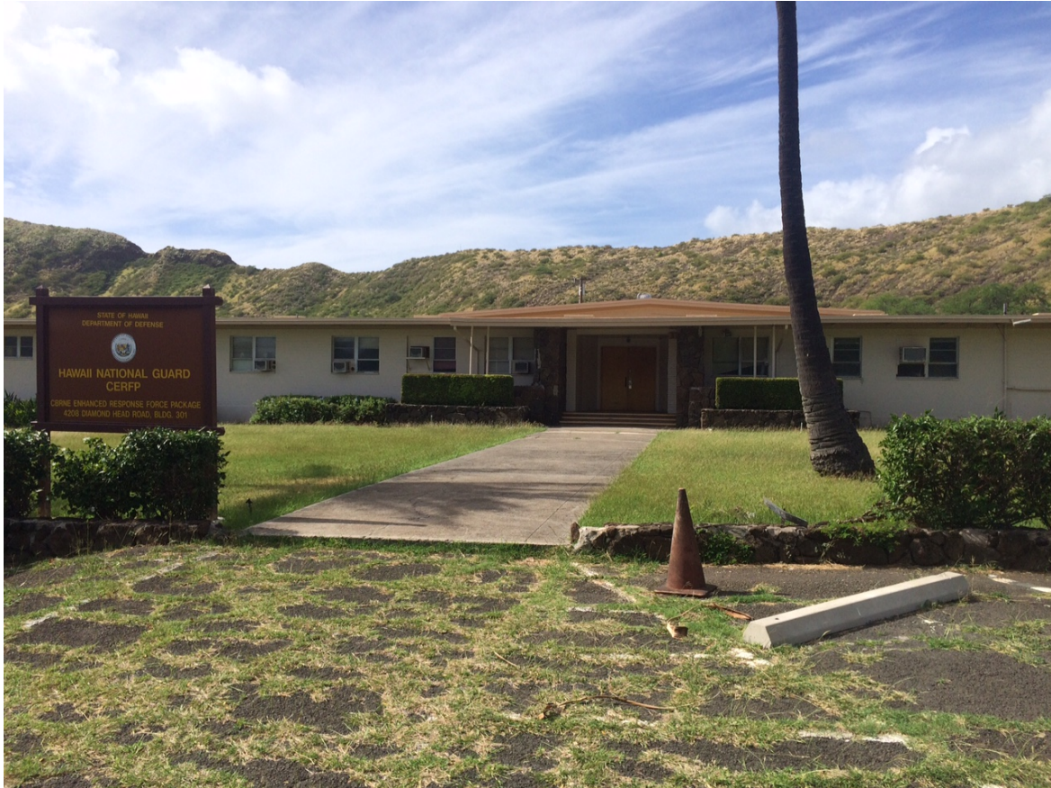
Bldg 301 Primary Facade
