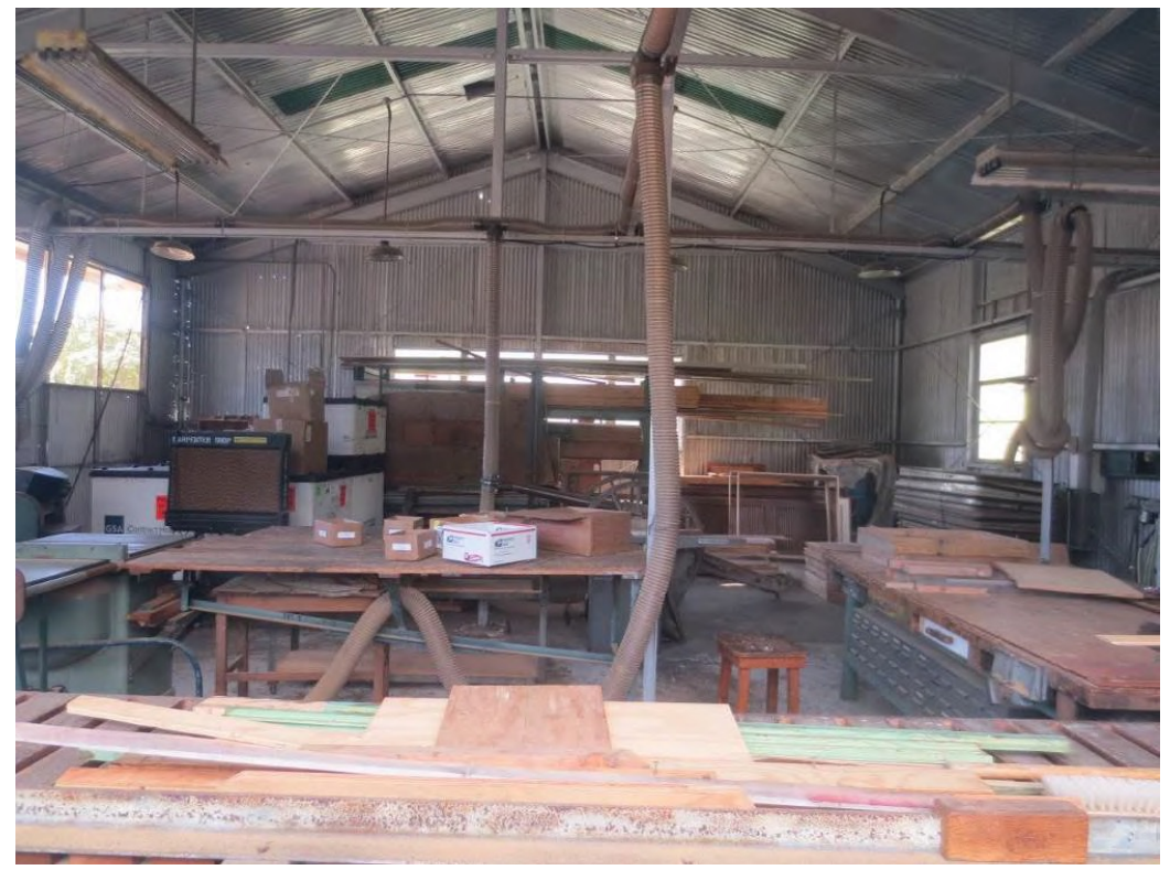
Bldg 304D Interior
