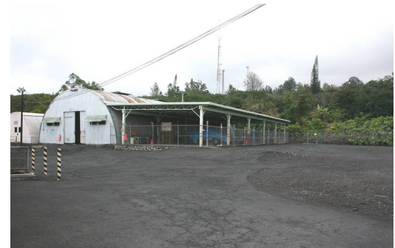
Kealahou – Vehicle Maintenance Shop. Built circa 1949.
