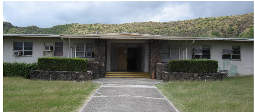
Bldg 301 Primary Facade
