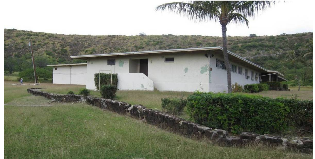
Bldg 301 Southwest Façade and lava rock wall
