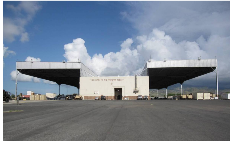
Kalaheo – Navy Maintenance Hangar. Built 1958.
