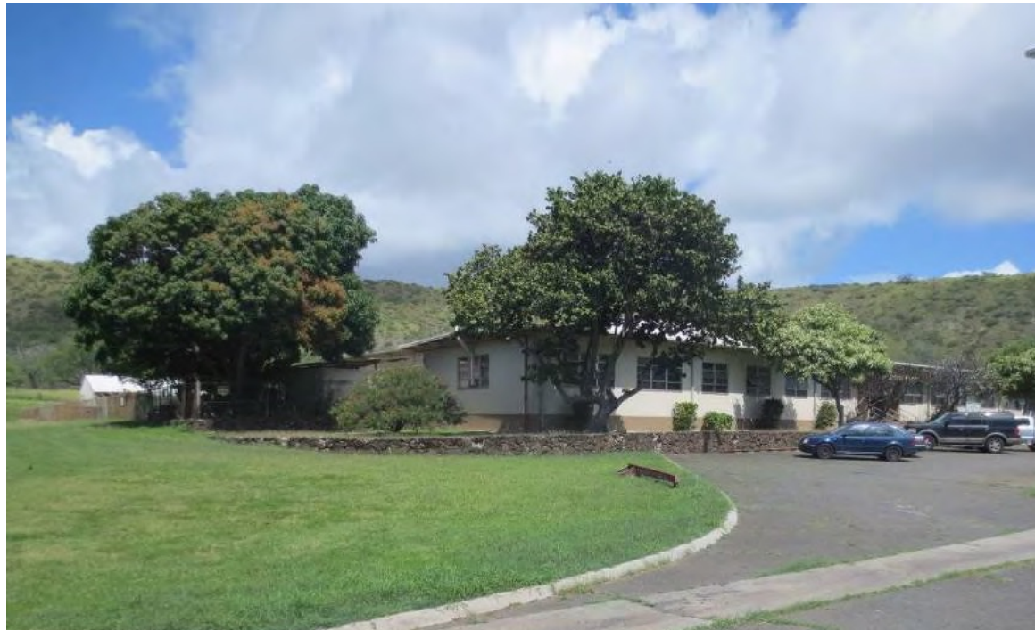
Bldg 304 Primary Facade
