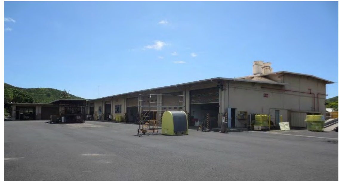
Bldg 304 Rear Shop Portion
