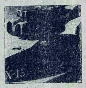
MOTHER'S WING--The experimental X-15 is shown just before it was dropped from the wing of a B-52 Stratofortress in a recent free-flight test over Edwards AFB, Calif. An F-100 chase plane can be seen in the background. (AFPS)
