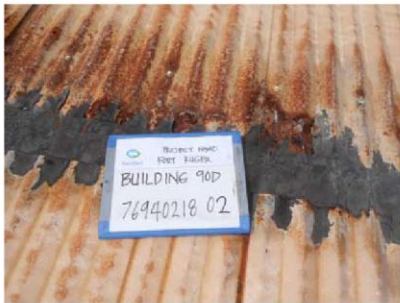
Photo 3: Building 90D. Non-asbestos containing black tar on the roof joint.
