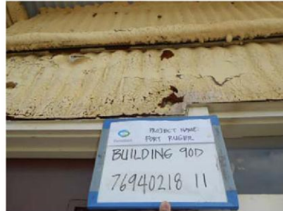
Photo 12: Building 90D. Asbestos containing black tar on the beige painted wall insulation.
