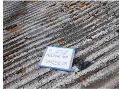
Photo 6: Building 90D. Non-asbestos containing black tar over foam insulation.
