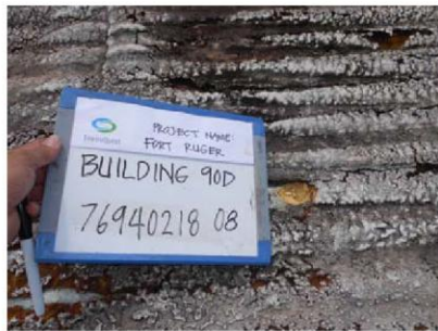
Photo 9: Building 90D. Asbestos containing roofing insulation black tar on the maintenance equipment roof.
