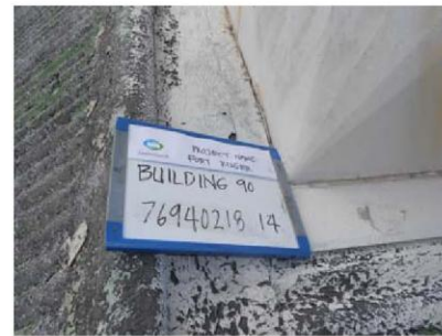
Photo 16: Building 90. Asbestos containing black tar sealant around the ventilator.
