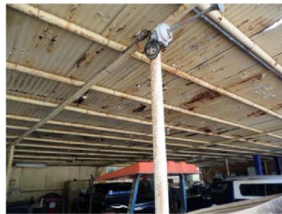
Photo 22: Building 90D. Lead-based painted cream metal carport post and roof frames.
