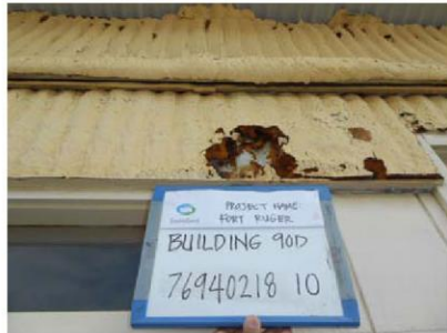
Photo 11: Building 90D. Asbestos containing black tar on the beige painted wall insulation.
