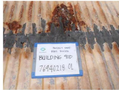
Photo 2: Building 90D. Non-asbestos containing black tar on the roof joint.
