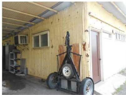
Photo 21: Building 90D. Non-lead based painted cream wall siding insulation and gray corrugated roof.
