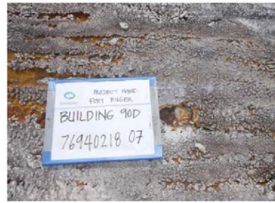
Photo 8: Building 90D. Asbestos containing roofing insulation black tar on the maintenance equipment roof.
