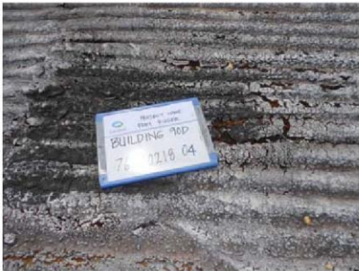
Photo 5: Building 90D. Non-asbestos containing black tar over foam insulation.
