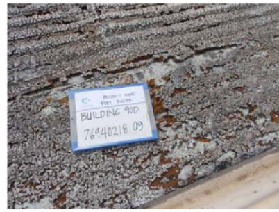
Photo 10: Building 90D. Asbestos containing roofing insulation black tar on the maintenance equipment roof.
