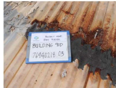
Photo 4: Building 90D. Non-asbestos containing black tar on the roof joint.
