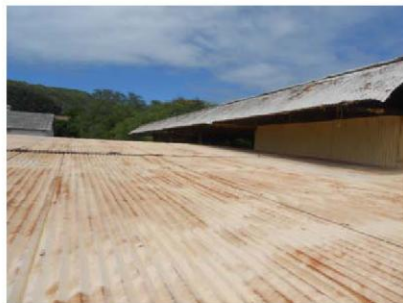
Photo 23: Building 90D. Non lead-based painted cream painted metal roof.
