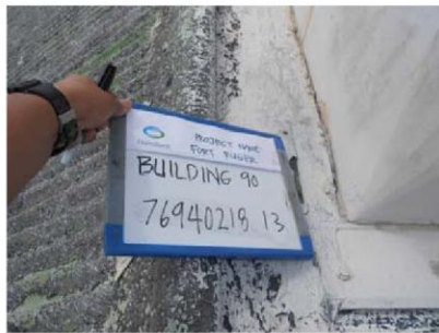
Photo 15: Building 90. Asbestos containing black tar sealant around the ventilator.
