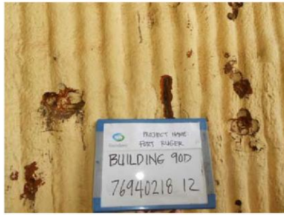
Photo 13: Building 90D. Asbestos containing black tar on the beige painted wall insulation.
