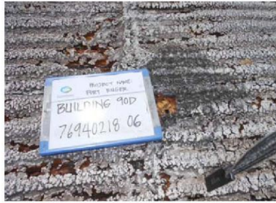
Photo 7: Building 90D. Non-asbestos containing black tar over foam insulation.
