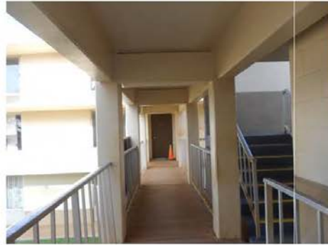
Photo 8: Hallway – concrete post, beams and deck. Lead-containing beige paint.
