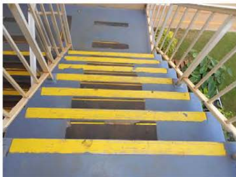
Photo 11: Staircase metal threshold. Non lead-containing yellow paint.
