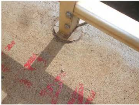
Photo 7: Hallway – aluminum post. Non asbestos-containing brown/gray concrete filler.
