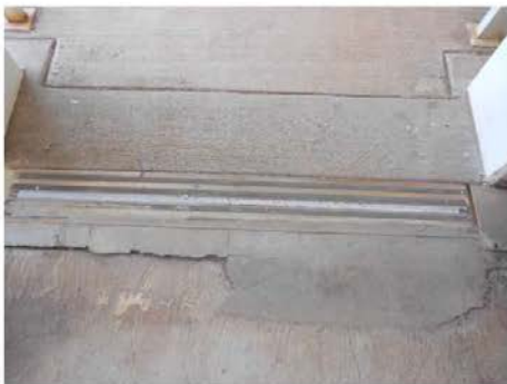
Photo 3: Hallway – floor expansion joint sealant. Non asbestos-containing gray caulking.
