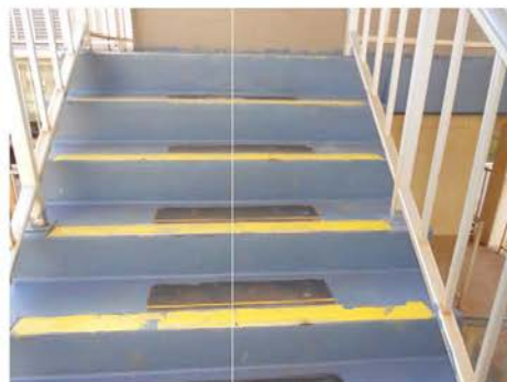
Photo 10: Staircase concrete steps and landing. Lead-containing blue over maroon paint.
