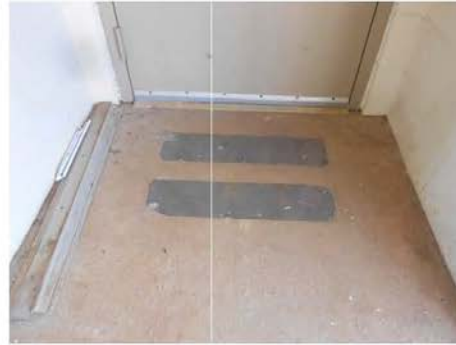
Photo 6: Hallway – adjacent to unit entry door. Non asbestos-containing black non skid paper and tan mastic.
