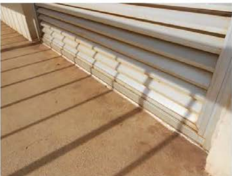
Photo 5: Hallway – floor and window louver sealant. Non asbestos-containing white caulking.
