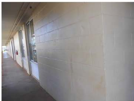
Photo 9: Hallway – adjacent exterior CMU wall. Non lead-containing beige over brown paint.
