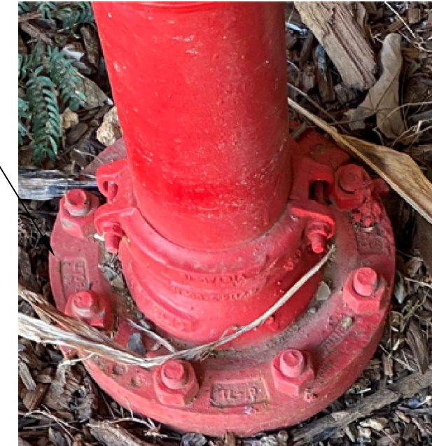
5 B711 CLASSROOM - EXST RISER CONDITION AT GRADE SCALE: NONE
