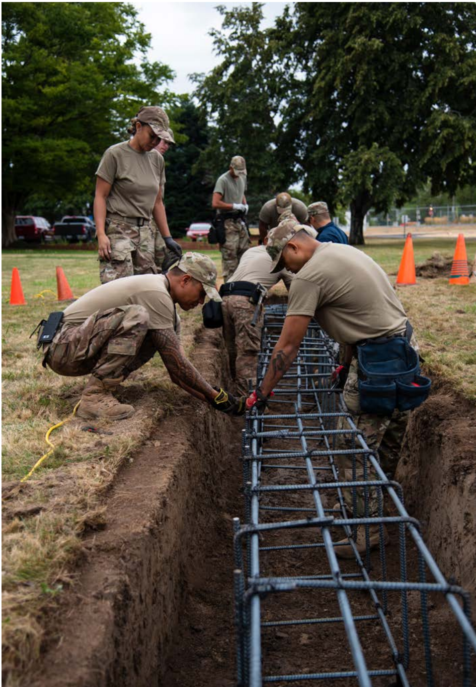
Members of the Hawai'i Air National Guard lay rebar in preparation for pouring concrete during annual training at Portland Air National Guard Base, Ore. on August 10, 2022. These Hawai'i Guardsmen are building a memorial wall as well as the foundation for a recruiting sign for the 142nd Wing during their two-week stay in Portland. (U.S. Air National Guard photo by Master Sgt. Steph Sawyer)
