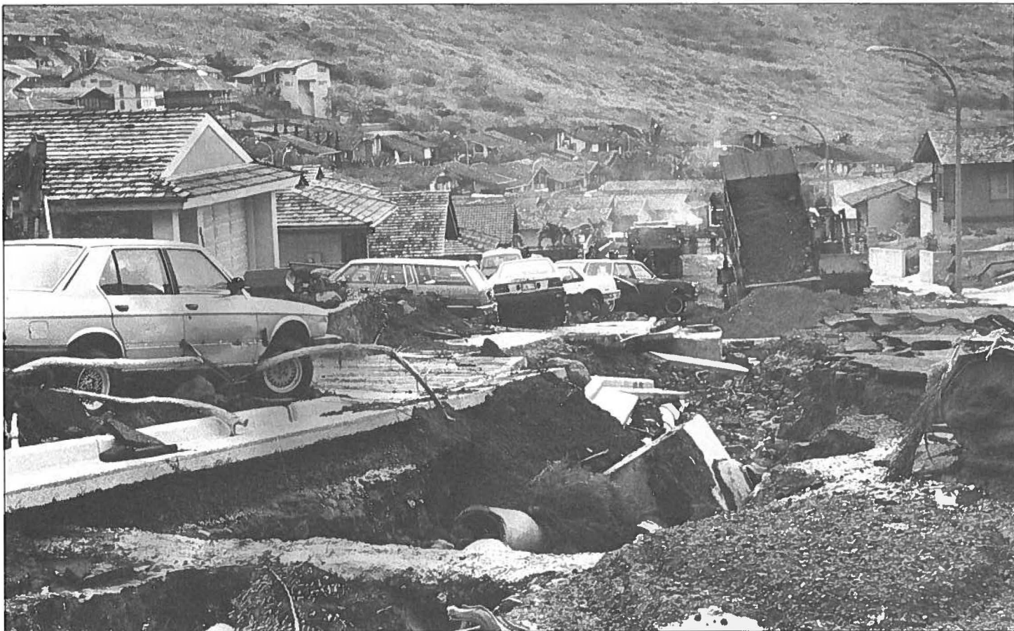
In the aftermath of Oahu's New Year flood, Hawaii Army National Guard dump trucks from the 227th Engineer Company brought in loads of dirt and gravel to repair the eroded Kahena Street. The temporary by-pass on Kahena Street enabled cars to be removed following the worst flood in Oahu's history.
