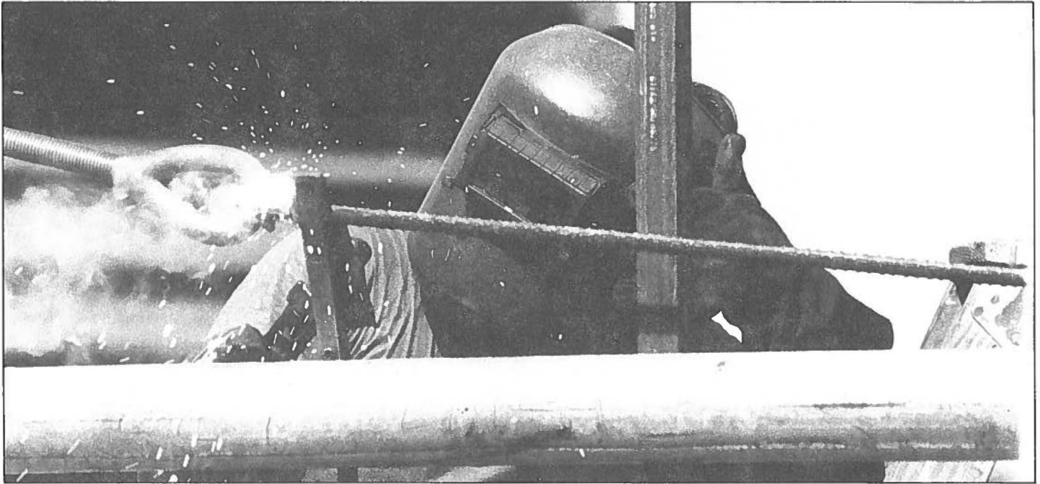
A 227th Engineer Company soldier welds a cable to the Kaena Point wild life refuge gate built to restrict access of motorized vehicles. The environmental enhancement project is Federal funded yearly.
