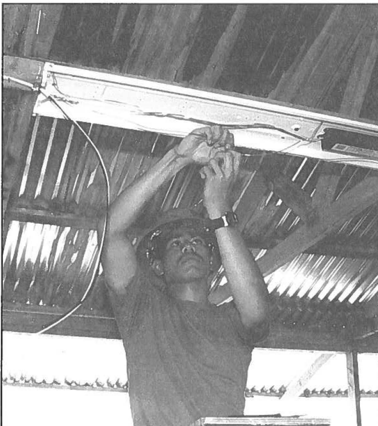
HOME IMPROVEMENT —Pvt. Nathan Taylau, an electrician with the 298th Engineer Detachment, wires the florescent light fixture in one of the newly constructed tropical huts in the Keaukaha Military Reservation in April 1998.
