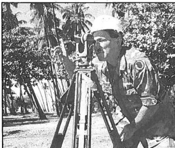
EVEN PLANE — Sgt. Vance L. Vidinha, 298th Engineer Detachment, directs the leveling of the area being prepared for the foundation of the new pavilion at Kalama'ulu Homestead's Ki'owea Beach Park, Molokai. 1st Lt. Jeffrey D. Hickman photo
