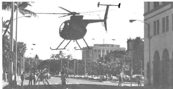
A helicopter was used to install a satellite ground communications station. CD telecommunications branch acts as technical advisors for the program.
