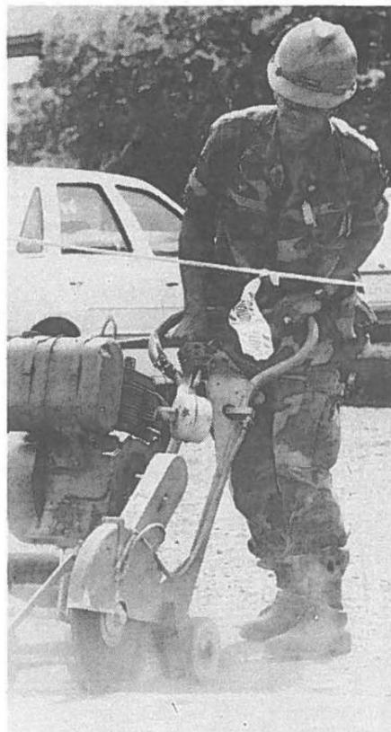
THE CUTTING EDGE—Sgt. Manuel Canoy, 298th Engineer Detachment, HARNG, cuts the asphalt, as he and other unit members dig a trench to bury an underground duct for power cables at the U.S.S. Arizona Memorial. (Photo by Sgt. Fred T. Kihara 117th PAD, HARNG)
