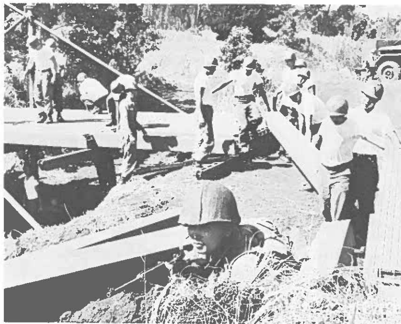
PFC Edwin Doiguchi, Co "B" 227th Engr Bn, stands guard while his company erects a M-4 Fixed Dry Span bridge with trestle.
