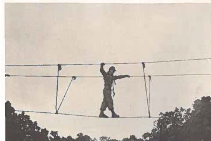
Three strand rope bridge is easiest to use, hardest to construct.
