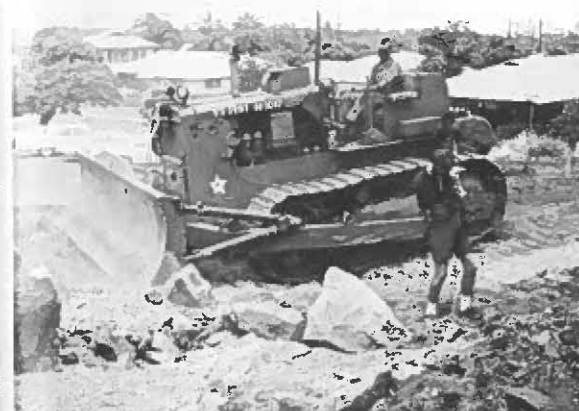
SURVEY —While SP5 Allan Hardy, 227th Engineer Company clears and grades the property adjacent to Ruger Theatre, Frank Herman, a volunteer worker for Honolulu Community Theatre, checks the grade. The 29th Brigade's Engineers assisted HCT in preparing the ground for construction of a new scenery and costume building.
