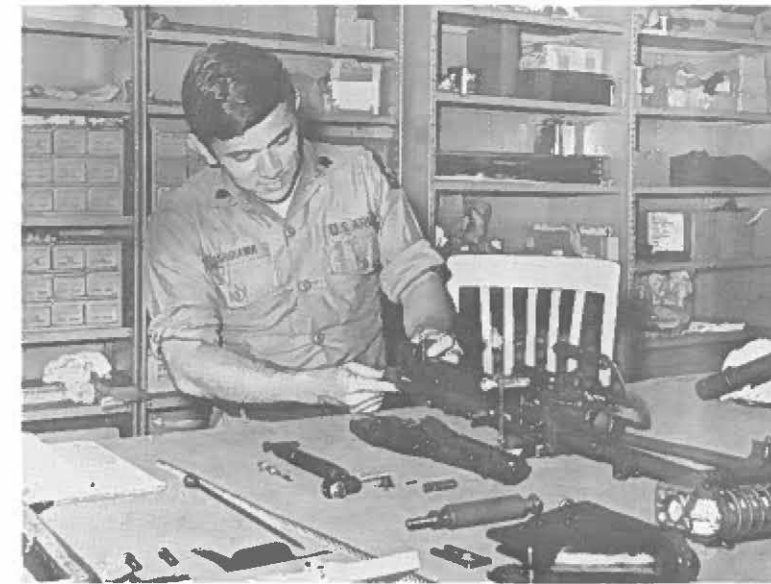
SP4 Ishikawa, an armorer, checks headspace on an M60 machine gun.
