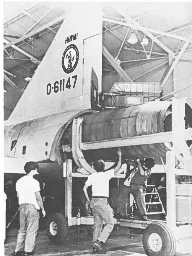
This is how the Air Guard pulls an engine.
